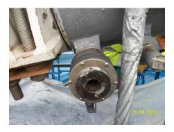
13.10 pm. Bolt "B" tightened up using hand pump to pressure as specified , pressure to be between 18,488psi and 19,578 psi.
