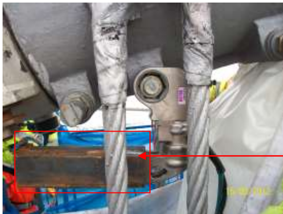
Extension sleeve fitted to RSL.6
