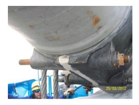
10.00 AM. Ps 4 applied to re-tension new bolt, pressure increments applied up to 16500 psi using air pump located on the footpath, this pressure was not enough to raise the tensioner to the acceptable required load as specified.
