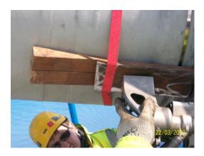
14.00 PM. Following no success in the use of this method, further discussions were held to offer an alternative method. Method adopted would require an extension sleeve to be fabricated and attached to the foot of the RSL 6 torque wrench. Engineer I. Alexander returned to workshop to complete proposed fabrication.
