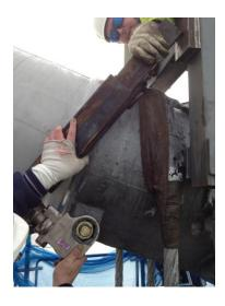
09.15 AM. Bolt "D" released . Slight coating of moisture was observed on bolt sleeve.
