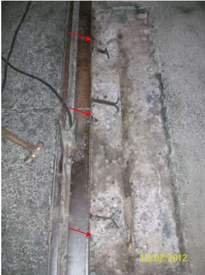
Existing Tangs, re-welded
