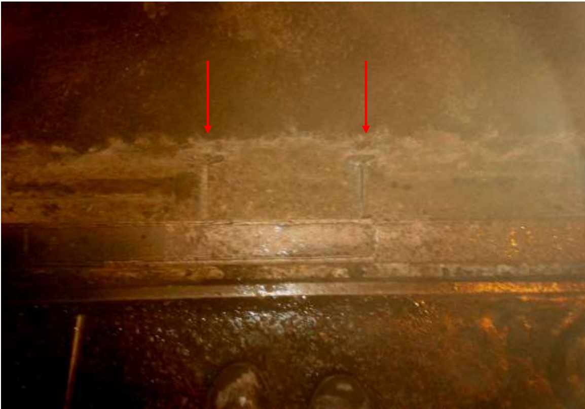
New Tangs welded into place.
