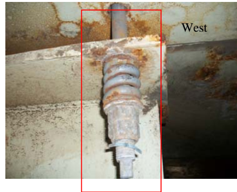
ME3 West Tongue plate spring, remains under tension no movement evident – post inspection.
