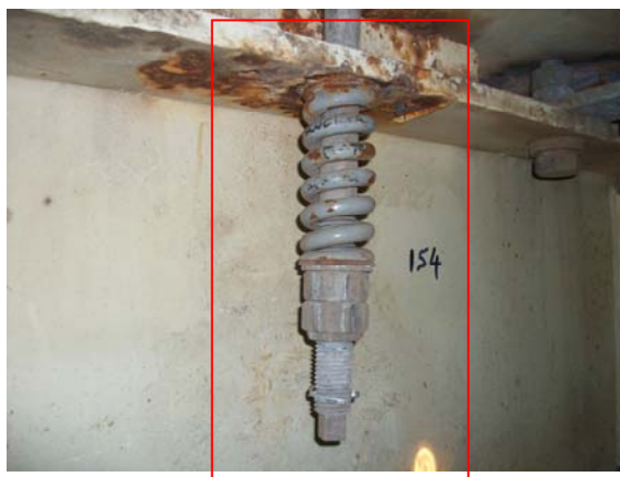
Rocker plate spring ME 3, remains under tension no movement evident – post inspection.
