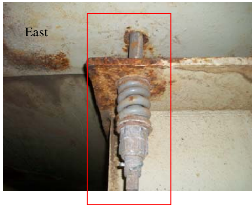
ME3 E East Tongue plate spring, remains under tension no movement evident – post inspection.
