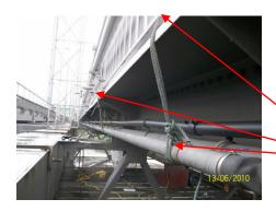
Section of service ducting being supported at 2 locations with rope over a distance of approx 6 mtrs. All holding / support brackets either missing or broken. Between PP69 & 71 east
