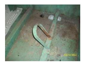
Located on the floor in section box 31x between outrigger beams 126/127 there is the original holding bracket for drain. (this will be removed by Balfour Beatty)
