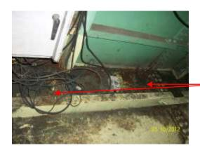
Floor section on the east side of section box 42x between outrigger beams 172/173 requires to be cleaned, also cables require to be tidied up.
