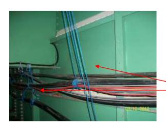
Located in section box 32x between outrigger beams 128/130 ducts/cables supported by ropes.
