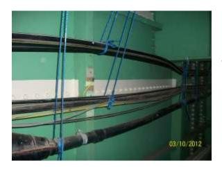
Located in section box 31x between outrigger beams 125/126 ducts/ cables supported by ropes.
