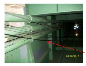
Cables located on the east face of box girder from section box 44x through box girder to section box 52x. require to be secured. Cables hanging down.
