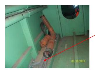
Located on the floor of section box 31x on the east side of the box girder between outrigger beams 110/111 cable tray / unistrut etc. (downpipe sections will be removed by balfour beatty)
