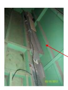
Located in section box 32x between outrigger beams 130 /132 cable tray / wires lying on floor.
