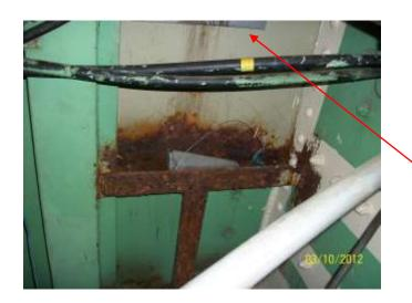
Egress for cables . water coming through cored holes in north east face. ( first reported 2004. requires to be sealed and corrosion cleaned up.
