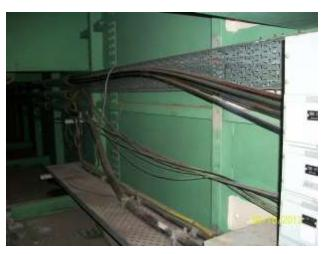
Cables located on the east face at section box 53 x between outriggers 219/222 require to be supported tidied up.
