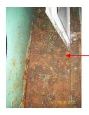
Floor section located in box 53x between outriggers 221/222 requires to be cleaned up staining /corrosion evident.
