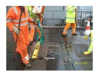
14.30- 14.40 .Bridge inspectors carry out and record Post removal dimensions of plate SE. 3.
