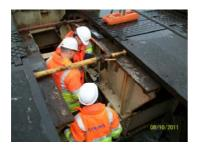
On completion of their visit, it was agreed that plates on ME 3. could be reinstated following the addition 10 mm packer plates under the Tongue plate to remove the mis-match between tongue plate end and bitumen plate
