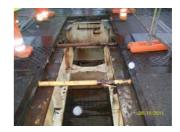
07.00 – 07.30. approx. Bridge staff cleaned both Tongue, Rocker & shuttle plates on ME3. by pressure washing. Cleaning of the radius arm girders and associated support and under-deck steelwork also carried out.
