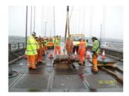
12.20- 12.35. Bridge staff cleaned both Tongue, Rocker & shuttle plates on ME3. by pressure washing. Cleaning of the radius arm girders and associated support and under-deck steelwork also carried out
