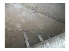
All Cycle track support beam slabs remain in very good condition both East & West. There are no signs of any longitudinal or transverse cracking or concrete spalling on any of the soffits of the beams. No evidence of any reinforcement movement, beam deflection or beam distortion at time of inspection.
