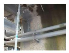
Side-span concrete corbel support blocks and top chord support columns.: All connection bolts and nuts have slight corrosion evident but remain in good condition, all remain secure and intact. All protection sleeves and welds remain in good condition. All attached side tower to top chord support columns both East and west remain in a satisfactory condition, although there is a small area of corrosion located on the north face, top west corrosion is evident.
