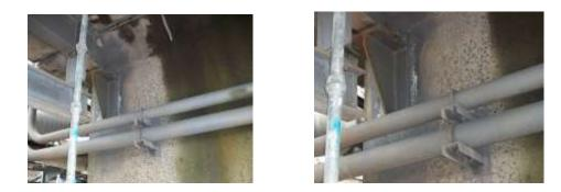
**D** & A line walkway support brackets (North face) side span side. Support brackets remain in a satisfactory condition on "A" line East & West and "D" line walkway connections to side tower. Plate location anchor bolts & nuts now showing signs of medium to heavy corrosion, No plate movement evident with all concrete in a satisfactory condition
