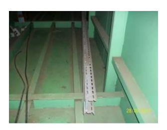
Photographs showing cable tray, unistrut, lighting boxes located in section boxes, for use in electrical program of works or removal.
