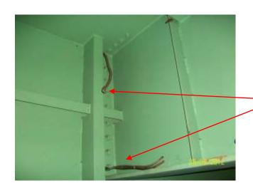
Located Between Outrigger Beams 104/105 in section box No 26, There Are What Appear To Be Redundant Cables Coming Through The East Face Of The Box Girder.
