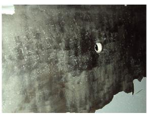
• 3.6 On many of the surfaces (exposed metal and/ or underside of paint flakes) which had been exposed for some time, it was noted that there was a thin film of yellowish grey-green contamination. Water swabbing had little or no effect on this material which was concluded to be non water-soluble and the discolouration that was lifted was presumed to be recent dirt.
