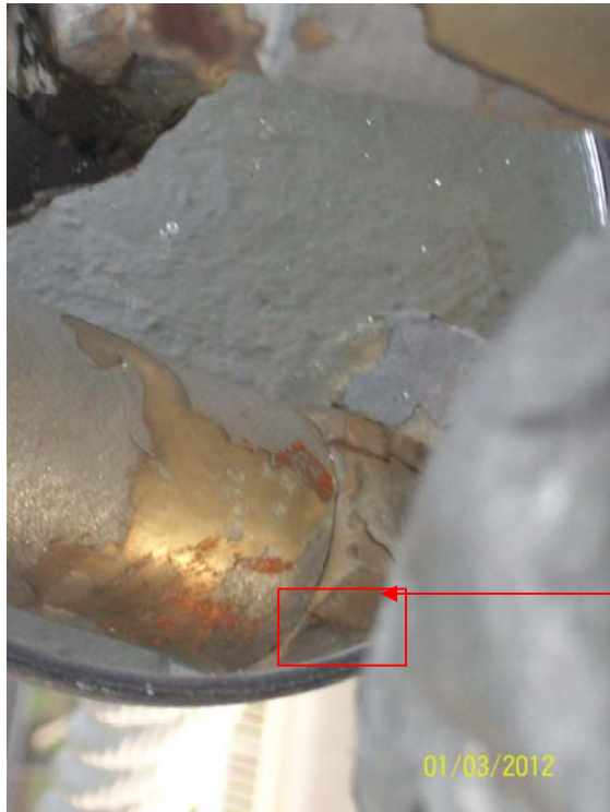
PP. 24. Bolt "D" Live side, nut crack recorded, bottom face.
