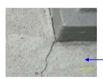
Paint crack leading from the S/E inner corner of the suspender casting to top chord at PP. 58 N/E.
