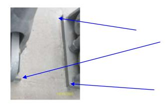
View showing paint cracks leading from all four inner corners of the suspender casting at PP. 58N/E.
