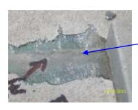
Ridge of metal on the top chord leading from the N/E inner toe of the casting plate. (paint removed) no sign of any defects.
