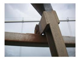
Sign Post Fold In Type Located On Handrail At Pp 80~N/E. Impact Damage Following Trailer Incident On 2014.07.29. Requires To Be Replaced . Work May Be Required To Top And Bottom Handrail Location Brackets. Slight Distortion Evident.
