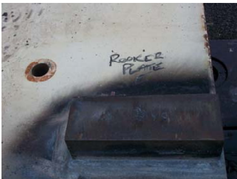
ME3 END BEARING BLOCK ON ROCKER PLATE (E) SHOWING WELDS CLEANED & TESTED.
