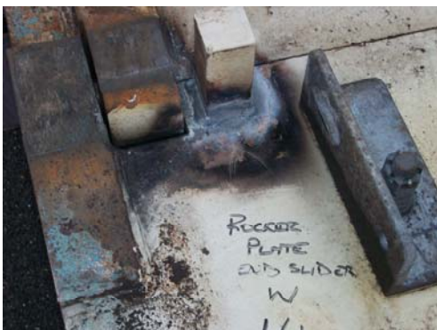
ME3 END BEARING BLOCK ON ROCKER PLATE (E) SHOWING WELDS CLEANED & TESTED.
