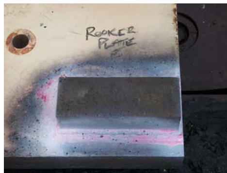
ME3 END BEARING BLOCK ON ROCKER PLATE (E) SHOWING WELDS CLEANED & TESTED.
