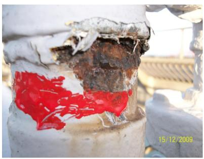
P.P.91 N.W. 2" AIR LINE TAKE OFF NIPPLE, IS HEAVILY CORRODED. RECOMMEND REPLACEMENT BEFORE PRESSURE LEAK
