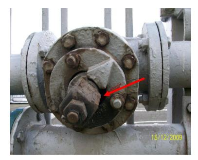
P.P.46 S.W. AUDCO VALVE PASSING AT VALVE STEM
