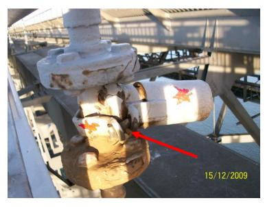
P.P.90 N.W. I" WATER VALVE HAS A LOOSE ANTI-TAMPER SLEEVE
