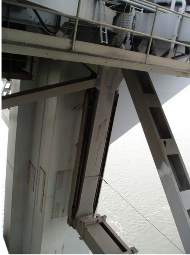
Figure 2 – Stiffening Truss End Post and Link
