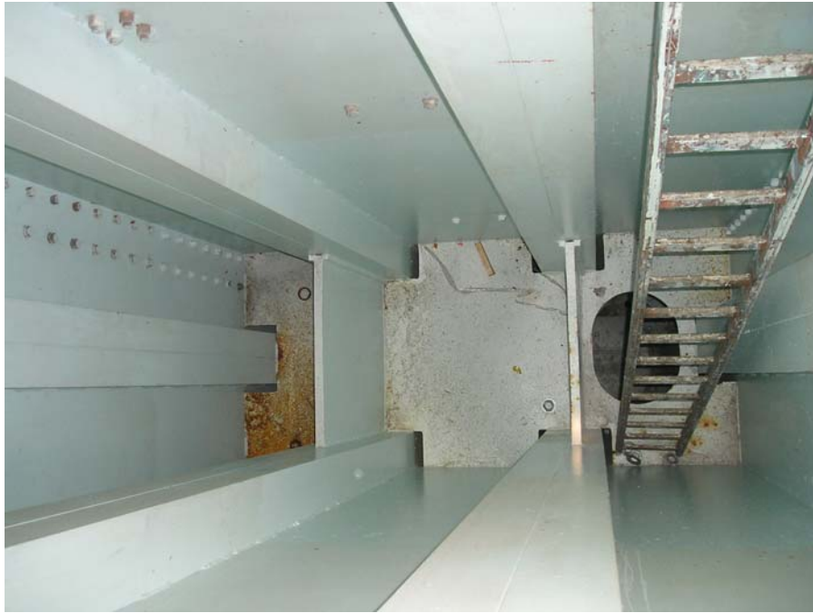
Figure 7 – View on bracket from within the tower, inner cell of the tower is topmost in the photograph
