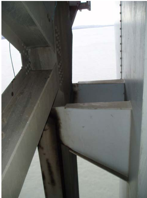
Figure 3 – Main Tower End Link Brackets
