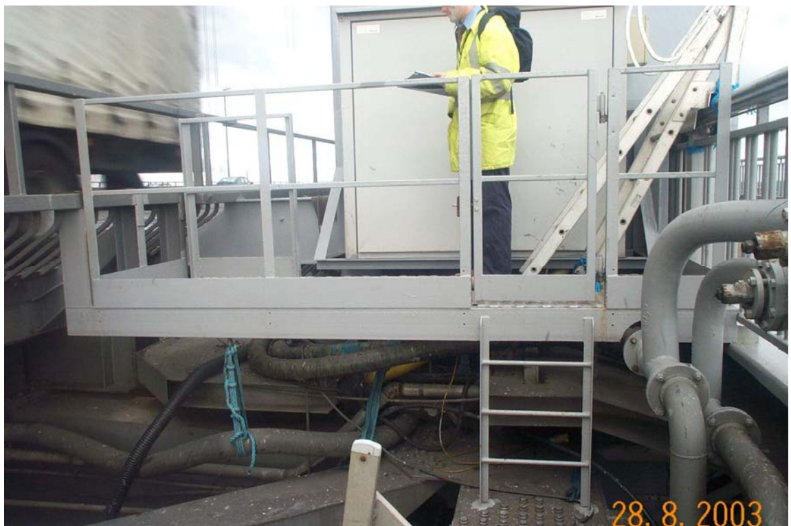
Figure 9 – Existing Electrical Distribution Box at Main Towers
