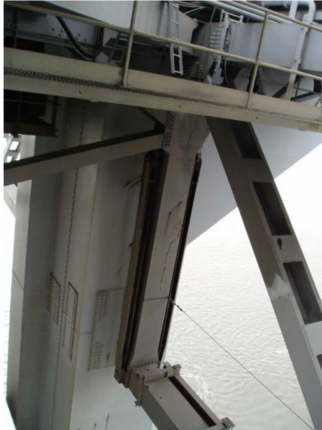
Figure 2 – Stiffening Truss End Post and Link
